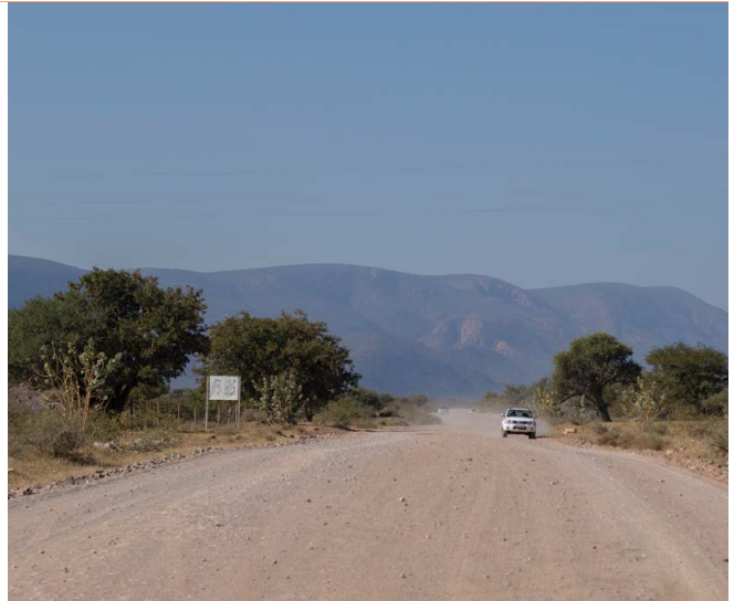
Road D3671, stretching from Musekwa to Maranikwe, is one of the gravel roads to be upgraded during the 2023/24 financial year.
