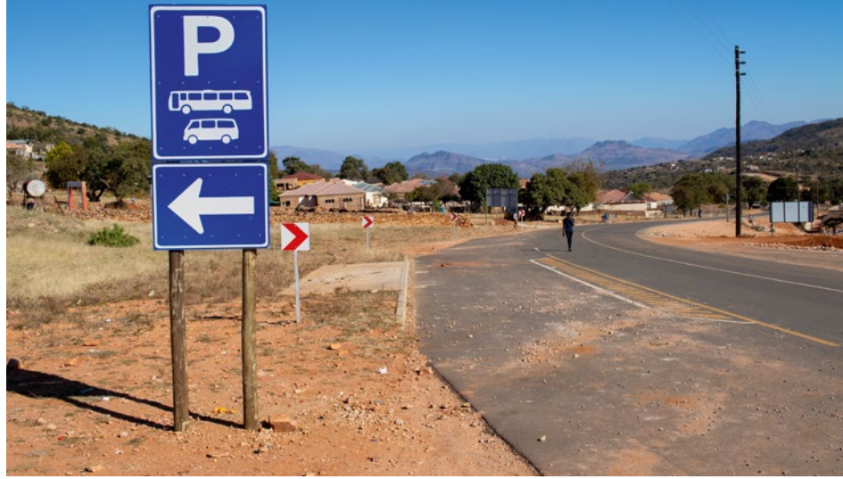
The Ga-Riba road project has made a significant contribution to many community members from the nearby villages who were employed as labourers.
