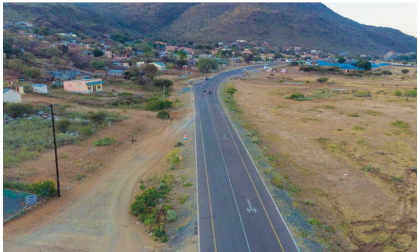
Limpopo Premier, Honourable Chupu Stanley Mathabatha, says since 1994 significant progress has been made in improving road infrastructure across the province, with most villages now having tarred roads.
