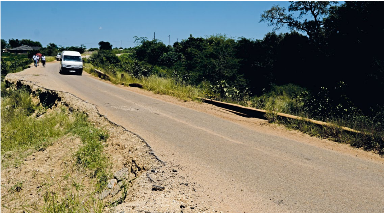
Makuleke Bridge before and after RAL intervention
