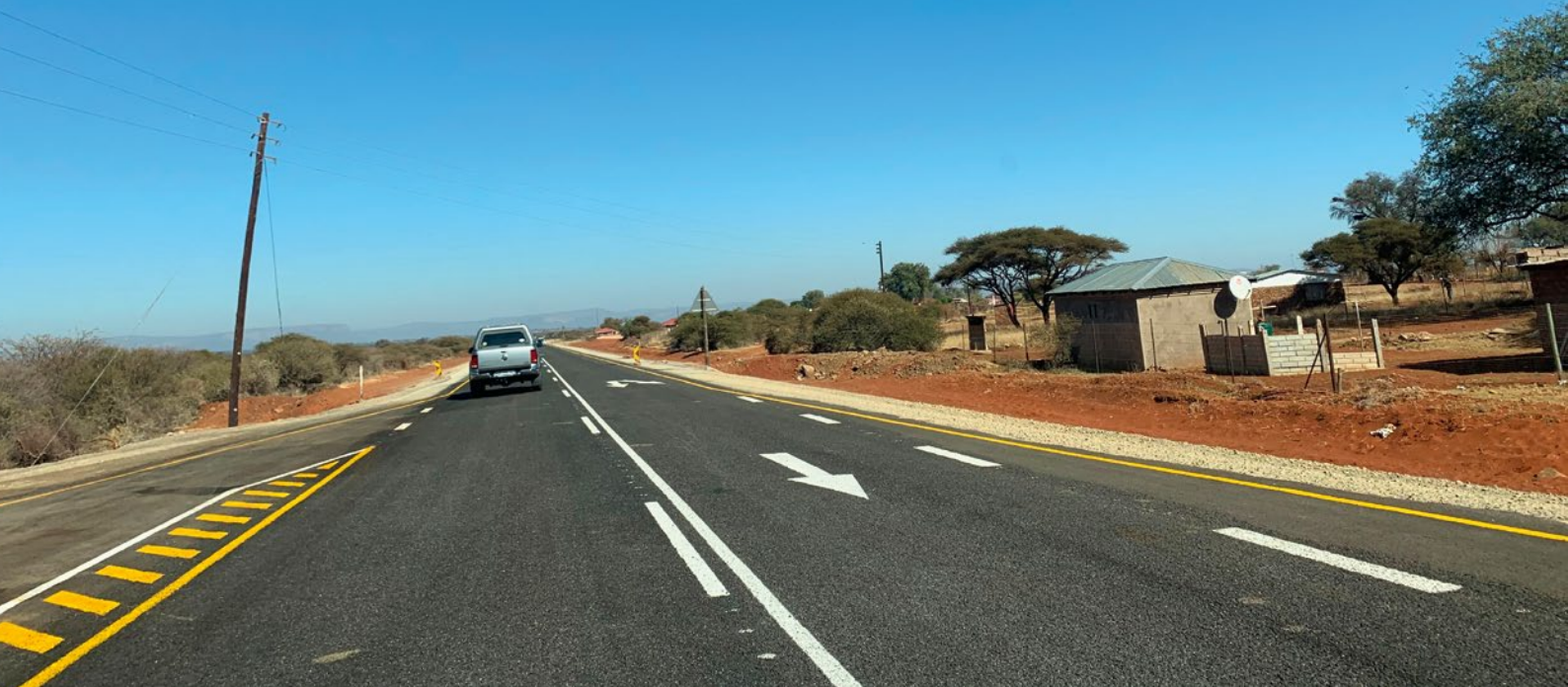
Road D3556 passing through the village of Tiberius in the Mogalakwena Local Municipality was constructed by community members recruited from up to twelve neighbouring villages. The road gives the community improved access to Tiberius Clinic.
